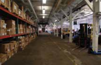
HD Supply Waterworks' New Britain facility has 12,000 sq. ft. of space, allowing virtually all inventory to be stored inside.
